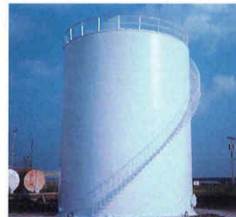
28' 6" x 32', 3,500 barrel fuel oil tank
