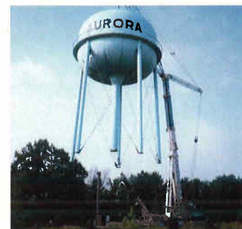
300,000-gallon municipal water tower. Raised 35 feet.
