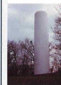
Above: 10' x 80', 100,000-gallon municipal water standpipe
