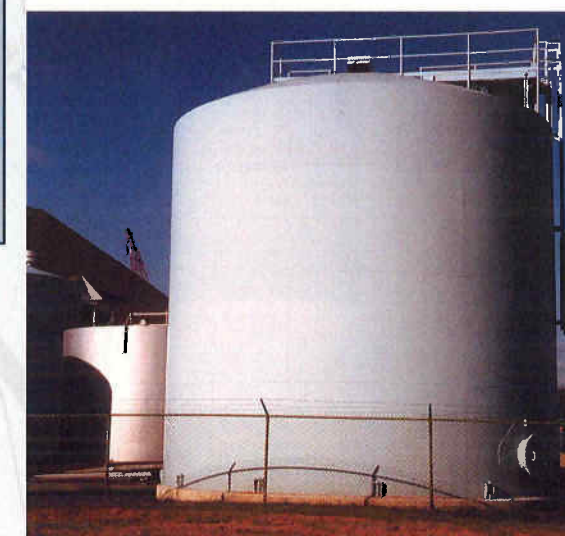
33' x 32', 200,000-gallon municipal water treatment facility
