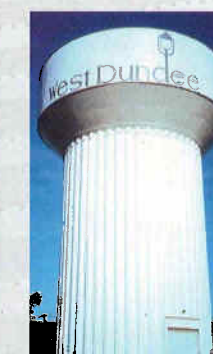
74' x 40', 1,000,000 gallon water treatment tank
