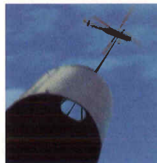
Above: 1,000,000-gallon municipal standpipe. Raised 30' to increase capacity and overflow elevation.
