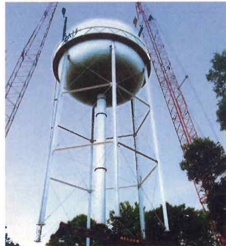
Above: 250,000-gallon municipal water tank. Raised 11'. Increased height to match existing system overflow elevation.
