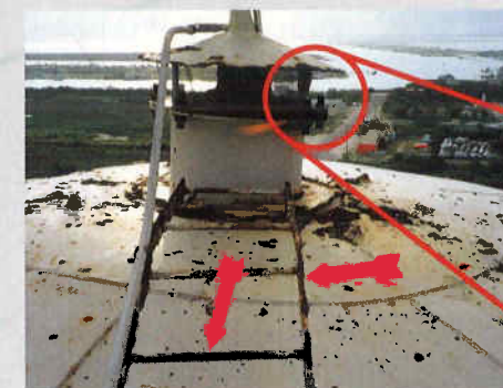
These photos illustrate the extent of severe damage found during inspections. Even this level of damage may be repaired. This dangerous severity, however, can be avoided with a proper maintenance schedule. The damage shown above and top right (on the vent) is especially easy to avoid, thereby preventing serious contamination potential.
