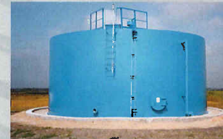
Left: 33' x 16', 100,000-gallon fire protection tank – industrial warehouse
