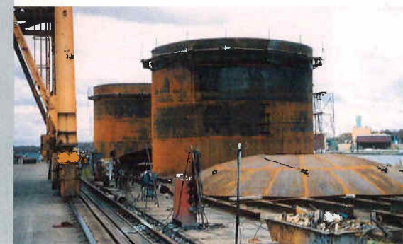
Two 40' x 30' fuel tanks in construction
