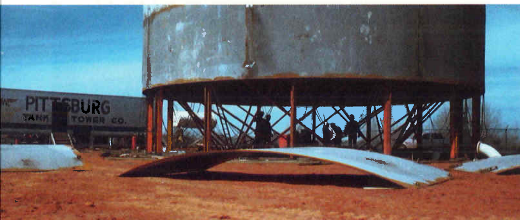
Above: 1,000,000-gallon municipal standpipe. Raised 30' to increase capacity and overflow elevation.
