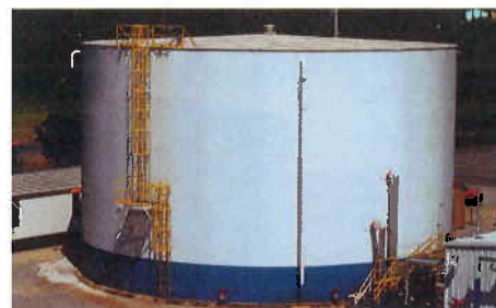
46' x 40', 490,000-gallon liquor storage – pulp & paper mill
