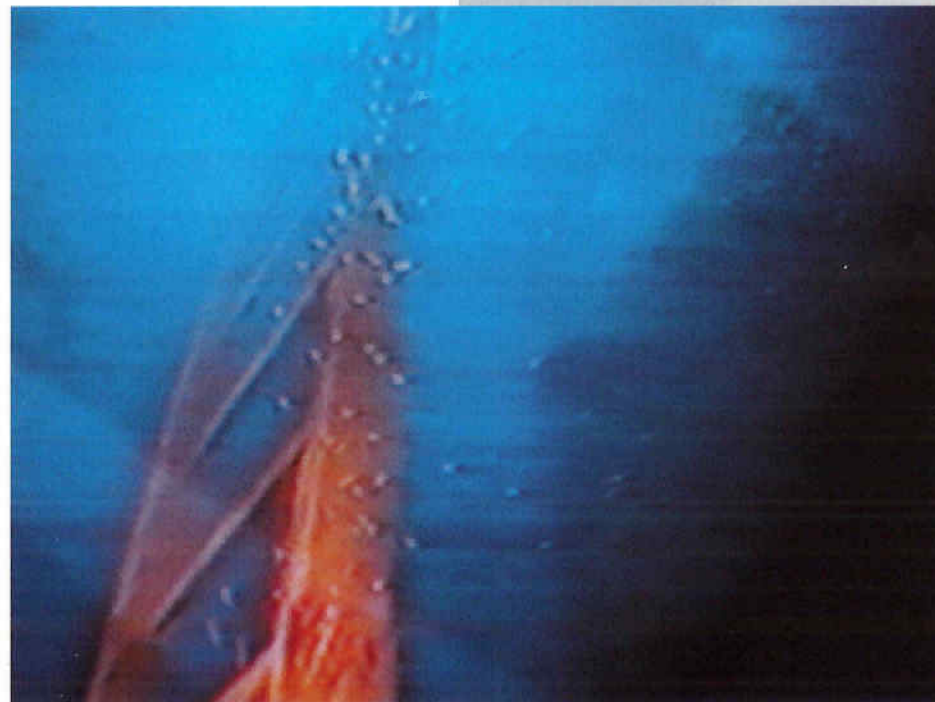
Above and Right: Underwater inspections are performed when a tank cannot be drained. Although this is not the preferred method of inspection, it is much better than delaying inspection. Minor repairs can be performed under water.
