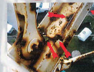
These photos illustrate the extent of severe damage found during inspections. Even this level of damage may be repaired. This dangerous severity, however, can be avoided with a proper maintenance schedule. The damage shown above and top right (on the vent) is especially easy to avoid, thereby preventing serious contamination potential.
