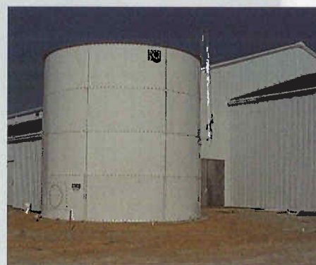
32,000-gallon municipal water bolted storage tank
